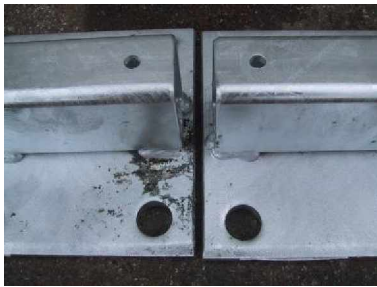
Damage of the zinc-coat due to unsuitable Anti-Spatter Spray (photo left), and unaffected after using METALLOTION PROTEC CE15L (photo right.)
